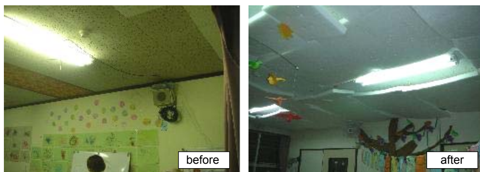
Figure 1: Installation of sound absorbing boards
